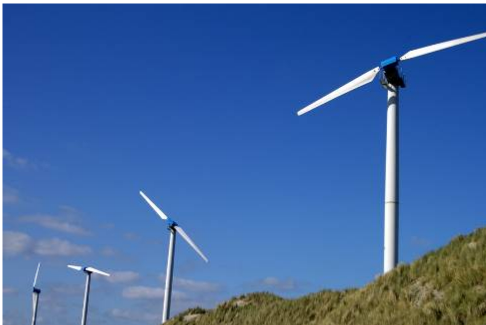
Four units on the Maasvlakte, the Netherlands
